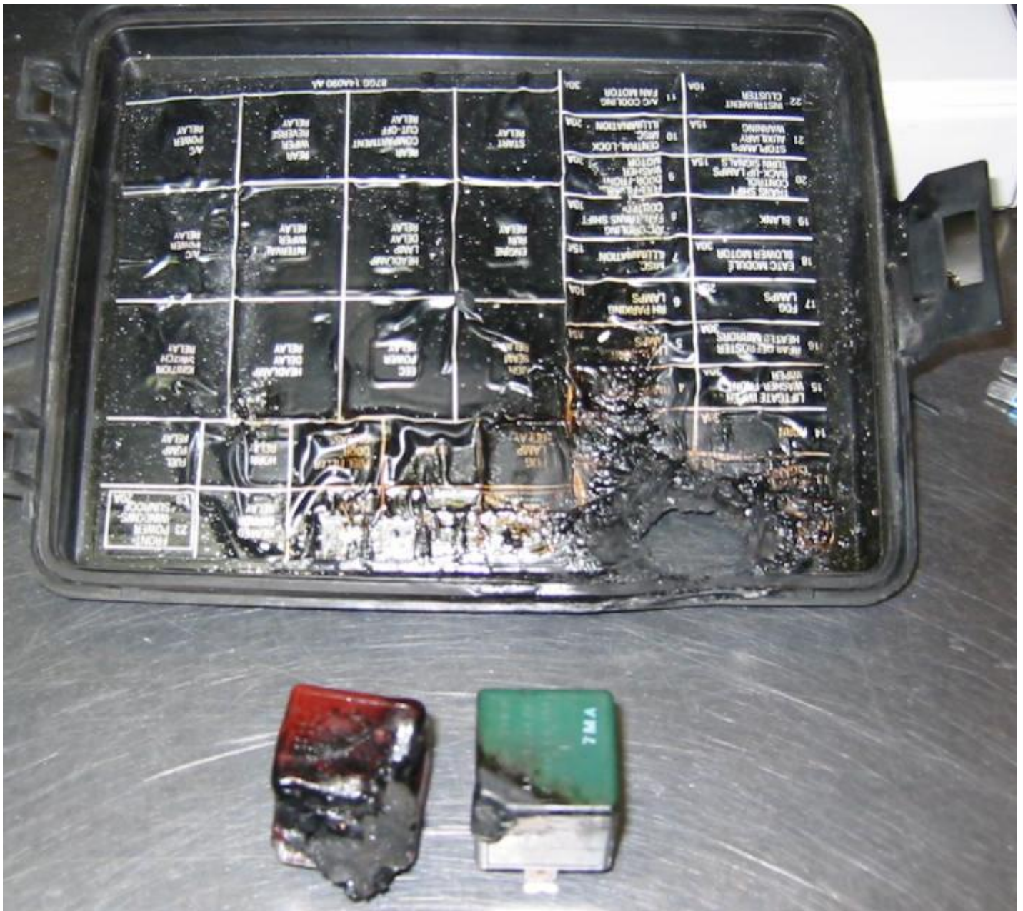
Here's the section of box I replaced. It took out three fuse holders- terminals and the plastic around them. I cut a section from another Scorpio fuse box, rather than replace the whole thing. It took a lot less time. I used a rubber piece on the far right side to patch the hole (the fuse box sits in a separate box). Seems to keep out the moisture.
